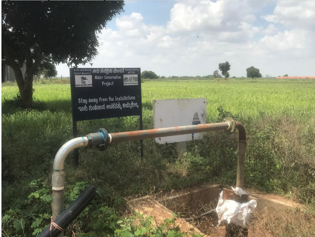
Figure 8: Recharge shaft at Nelamangala
